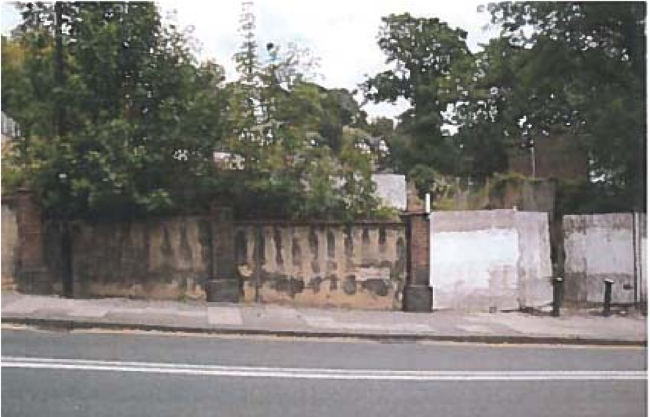
Front of site and remaining front boundary wall
